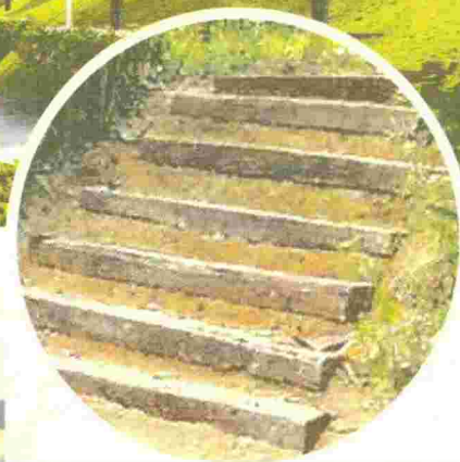
'Sleepers' from the Electrification of Double Track Project (EDTP) in the northern region.
