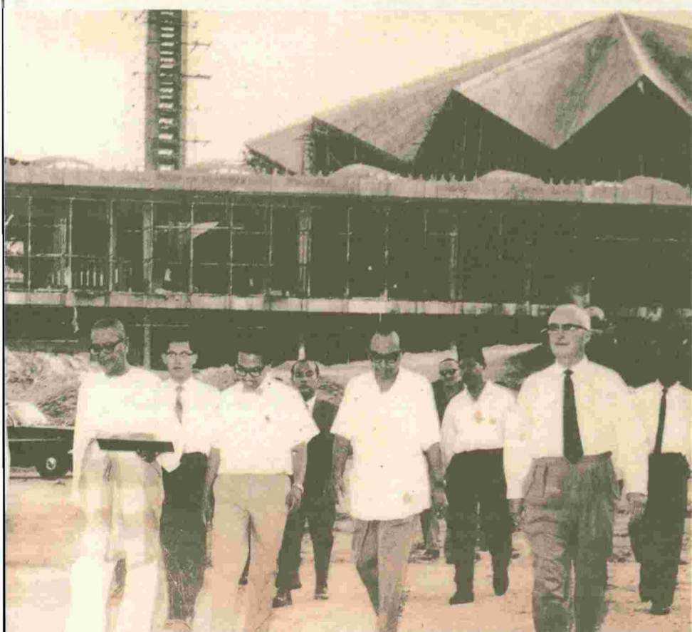
The site inspection of Masjid Negara by Tun V. T. Sambanthan (fourth from left) and Tunku Abdul Rahman.
